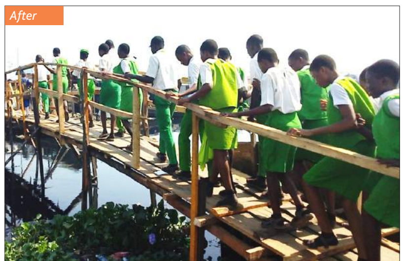
Students of Fazil Omar walking through the completed bridge constructed as part of their change project initiative
